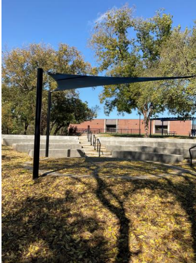
SAIL SHADE STRUCTURE AT AMPHITHEATER
